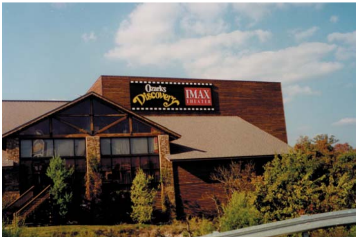
IMAX: Branson, Missouri chooses high tech jet induction diffusers and cold air distribution for occupant comfort.
